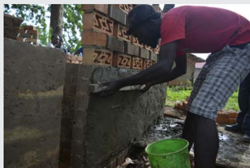
Cement-free plaster is added to protect the unfired bricks from surface moisture.
