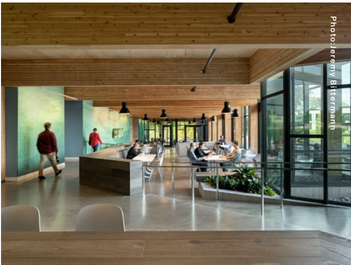
First Tech Federal Credit Union includes a 12×32-ft grid with 5-1/2-in. CLT panels spanning 12 ft between glulam beams.
